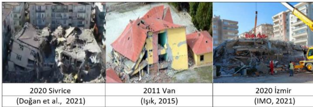
Figure 7. Destruction of (Grade 5) RC buildings
