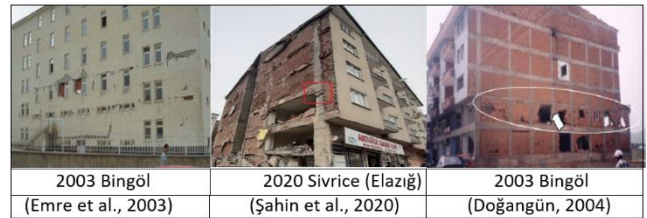
Figure 4. Moderate damaged RC buildings
