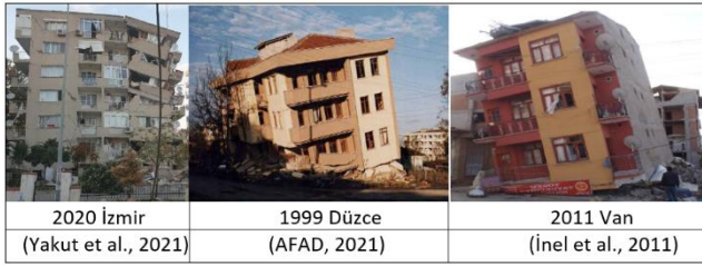
Figure 6. Very heavy damaged (Grade 4) RC buildings
