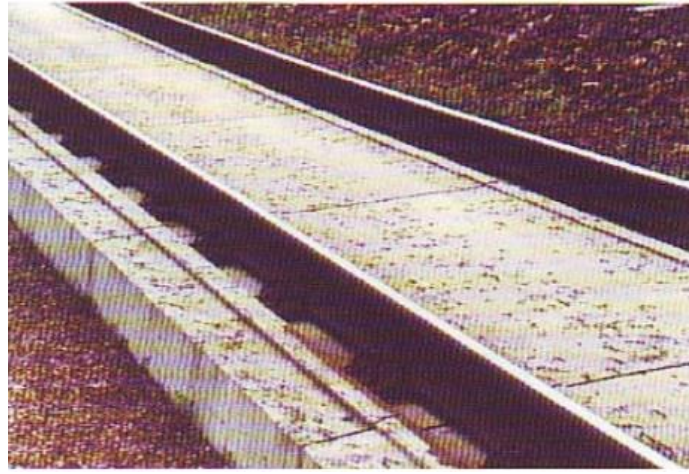
Figure 6. An example of a monolithic slab track design with direct rail fastenings (Esveld, Modern Railway Track 2nd Edition, 2001)
