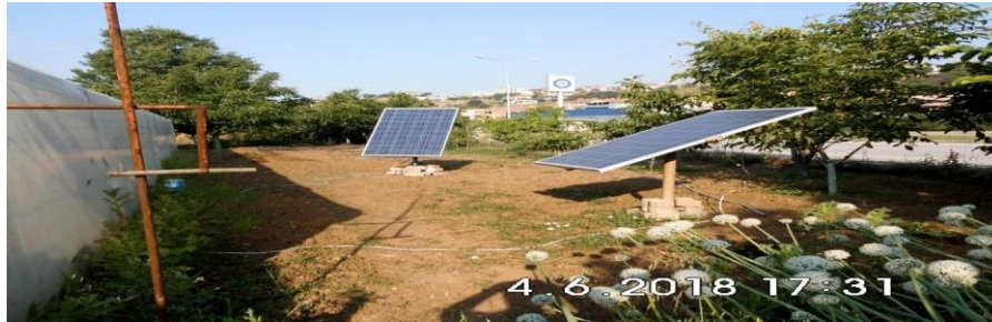
Figure 4. Solar panels; fixed and movable were mounted on a structure
