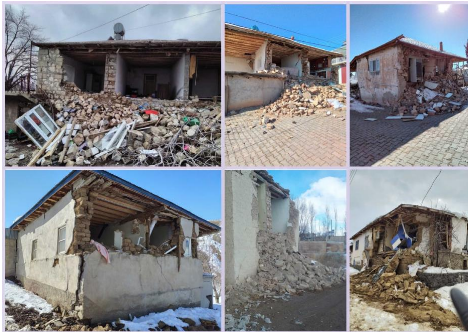
Figure 10. Example of out-of-plane movement on load-bearing walls
