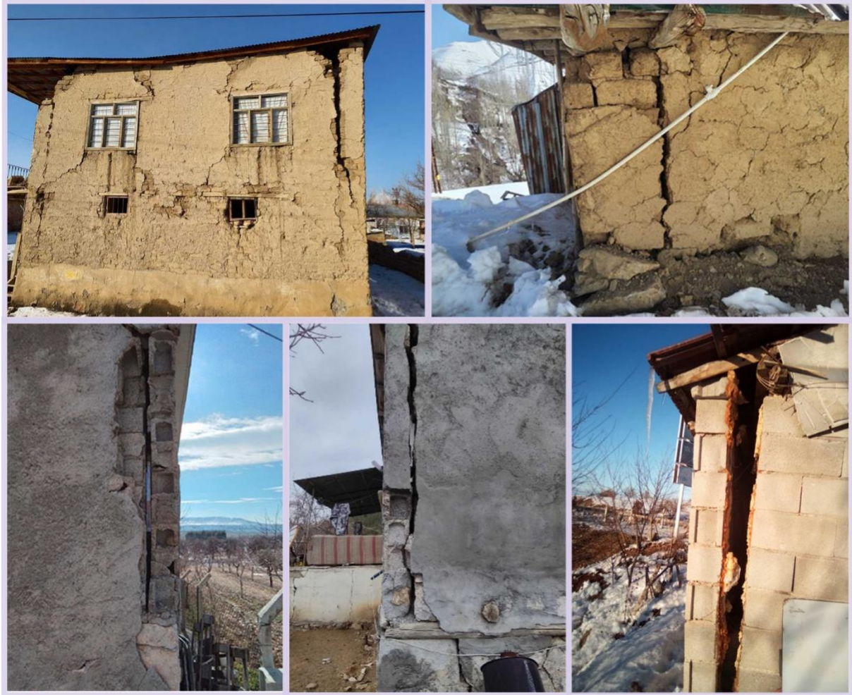
Figure 6. Wall separation at corners of the structures
