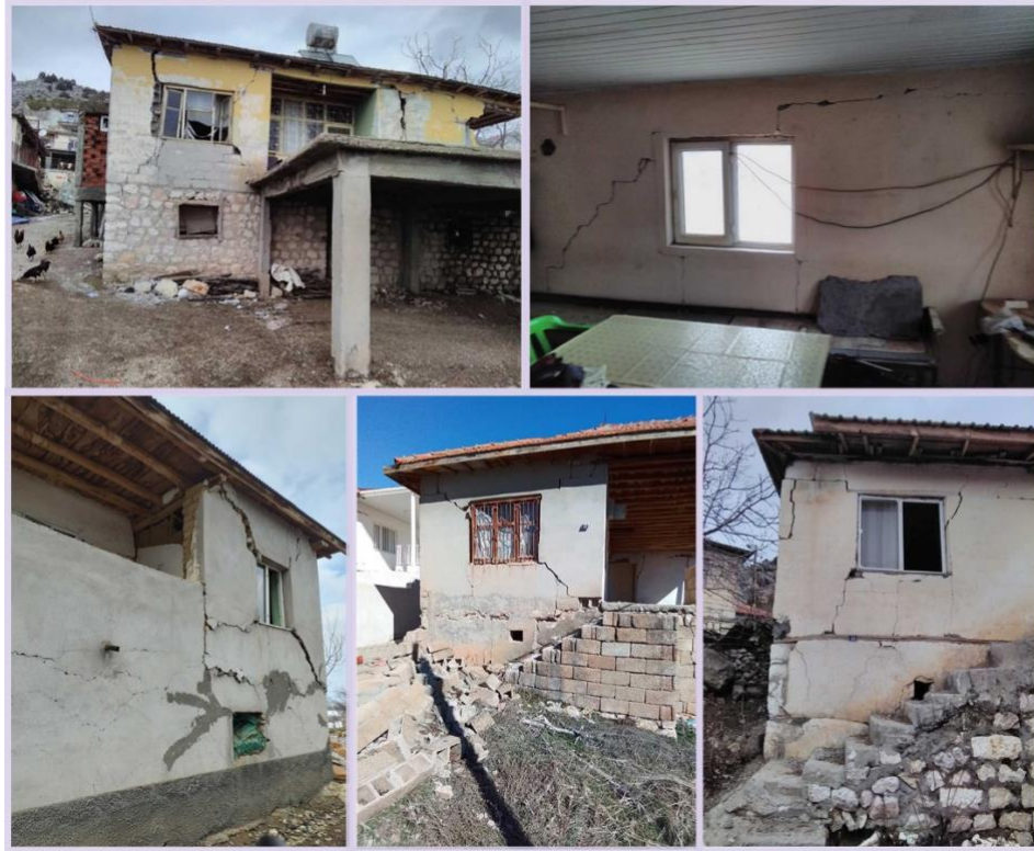
Figure 7. Damages at window corners
