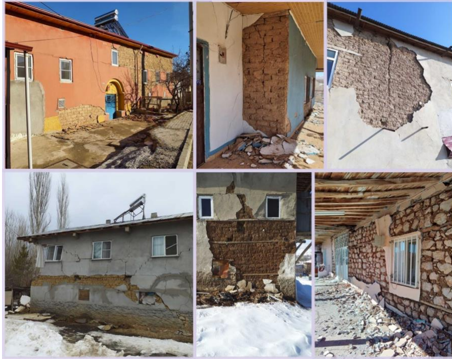
Figure 9. Falling of exterior materials
