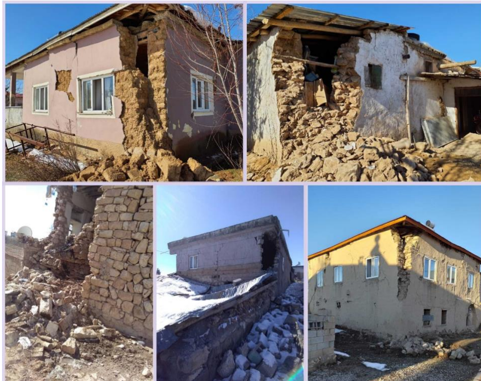
Figure 8. Examples of out-of-plane wall corner damage
