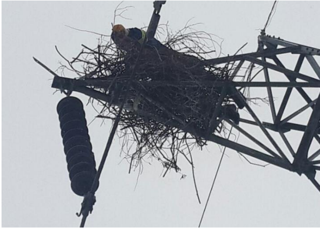
Figure 5. The Fault in 154 kV Tatvan-Muş Line
