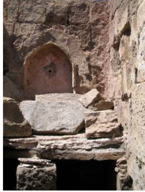
Figure 3. The water pipe and halvet niche
