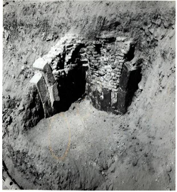
Figure 10. The squinch and the bricks which annihilated because of atmospheric conditions [5].
