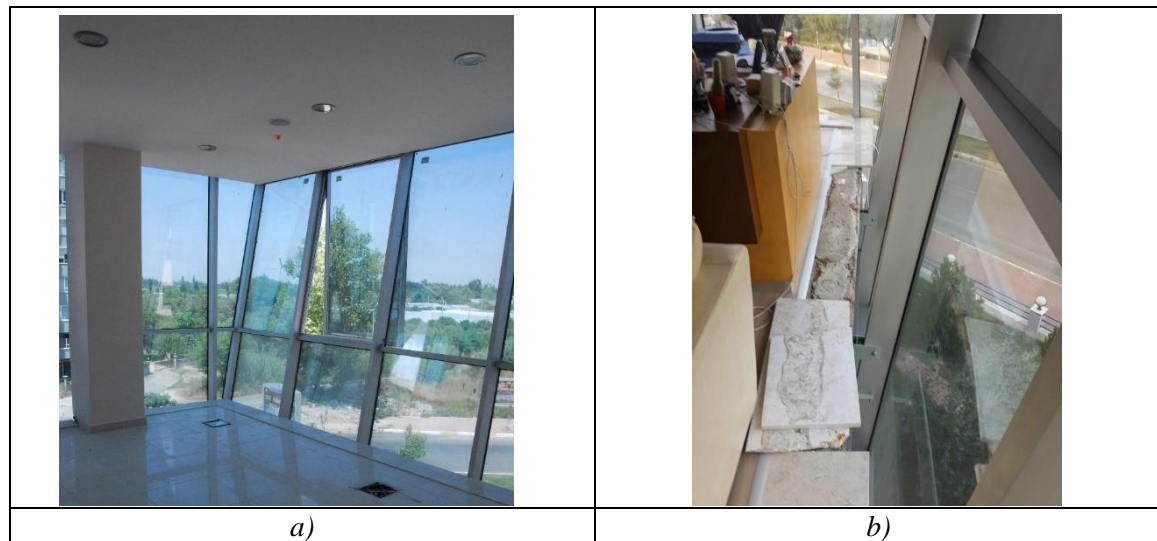
Figure 3. Photographs of GCW system from interior figure; a) View of the GCW from the interior ample b) Detailing of the GCW which leads to heat exchange between the floors
