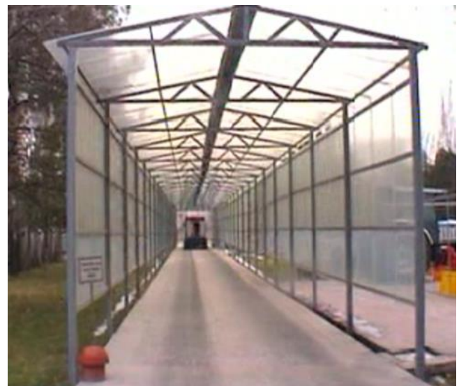
Fig. 1. Drawbar test tunnel
