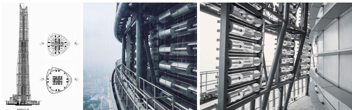
Figure 5. Section, plans and wind turbines, Shanghai Tower [19]
