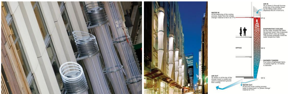
Figure 6. Use of rain tower, Council House 2 [12]
