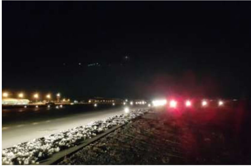
Figure 9. PAPI Light appears in different colors at different heights
