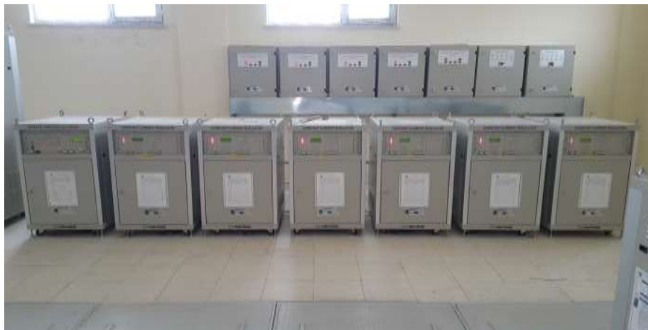
Figure 14. Constant current regulator in transformer building
