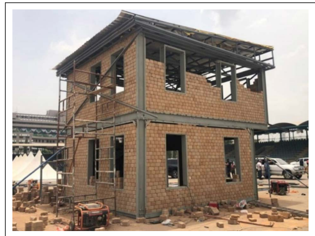
Figure 3. The ongoing building construction using ICSEB.
