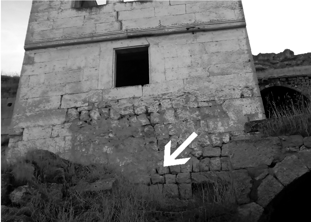
Fig. 12 Foundation type 4a: Deep-slope foundation
