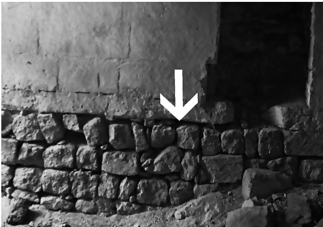
Fig. 13 Foundation type 4b: Deep-inner foundation
