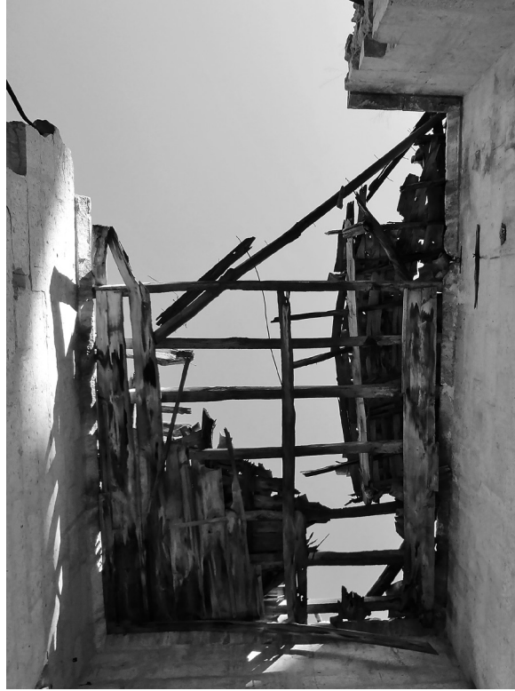
Fig. 23 Timber beams and ceiling coverings, bottom view
