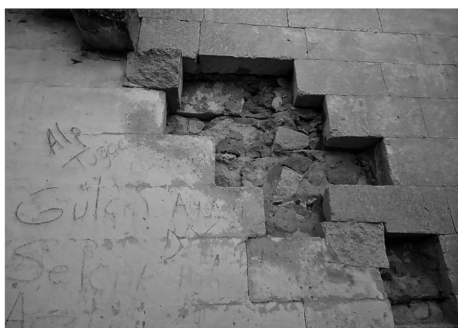
Fig. 17 Wall type 2: Thin, double- sided wall
