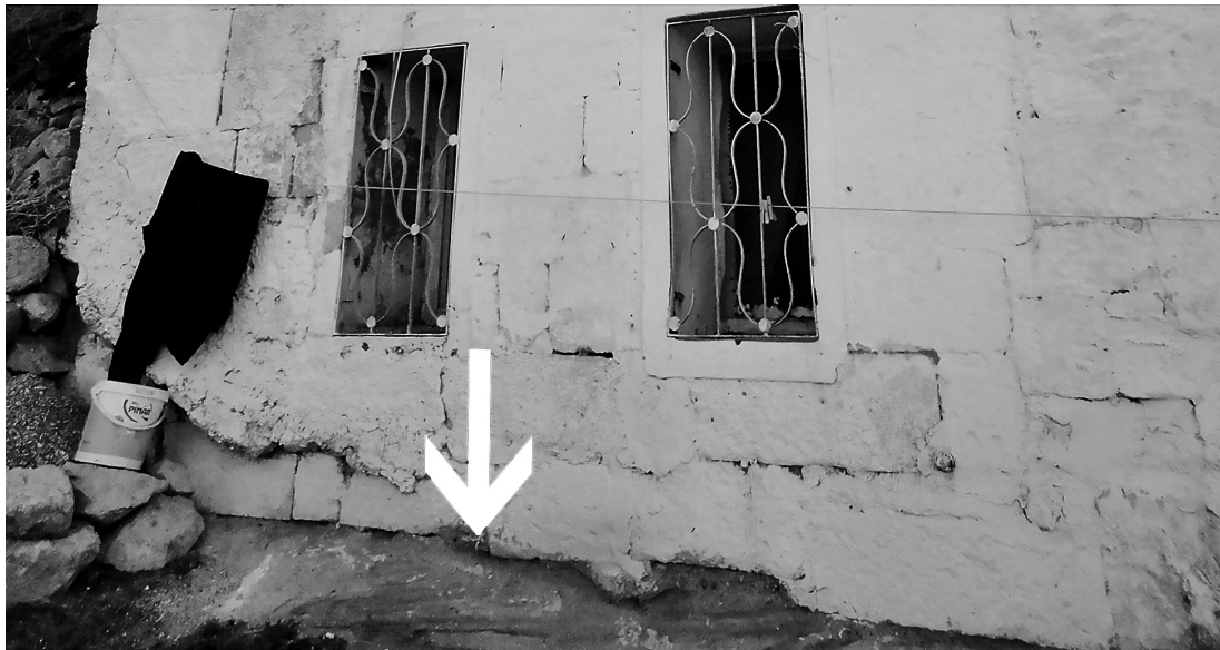
Fig. 11 Foundation type 3b: Shallow-inner foundation
