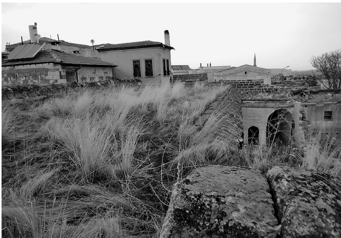
Fig. 26 Detail of earth roof
