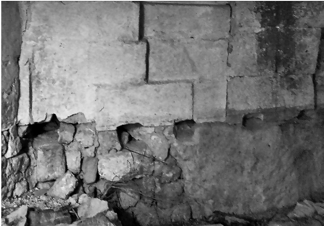
Fig. 8 Foundation type 1: Rock foundation
