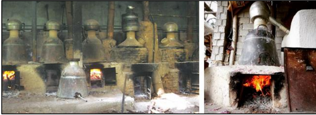
Figure 6: Boiling of Boilers.
