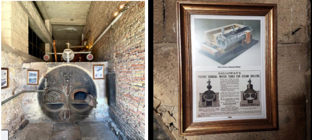
Figure 26: Güneykent Rose Oil Factory Historical Steam Boiler.
