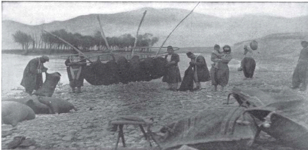
ARMENIANS CONSTRUCTING A RAFT OF INFLATED SHEEPSKINS ON THE BANKS OF THE EUPHRATES RIVER
