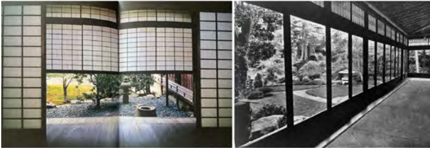
Figure 3. Shoji window and panel (translucent panels) (Takeshi, 2005), Engawa (veranda) (Yoshida, 1955)
