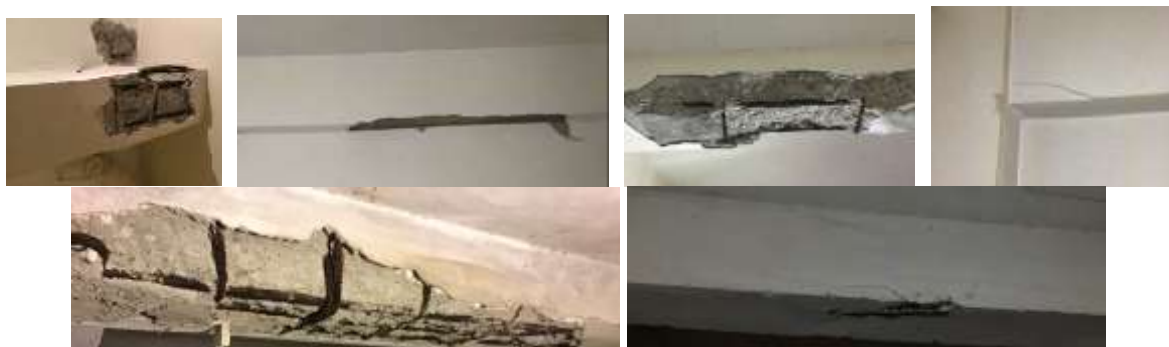
Figure 1. Images of corroded RC beams
