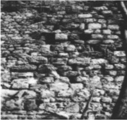
Figure 24. The cavities in “i” section tower II
