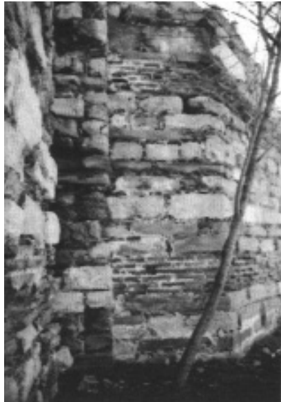
Figure 20. The brick courses end at the corner where walls “e” and “d” of tower II meet
