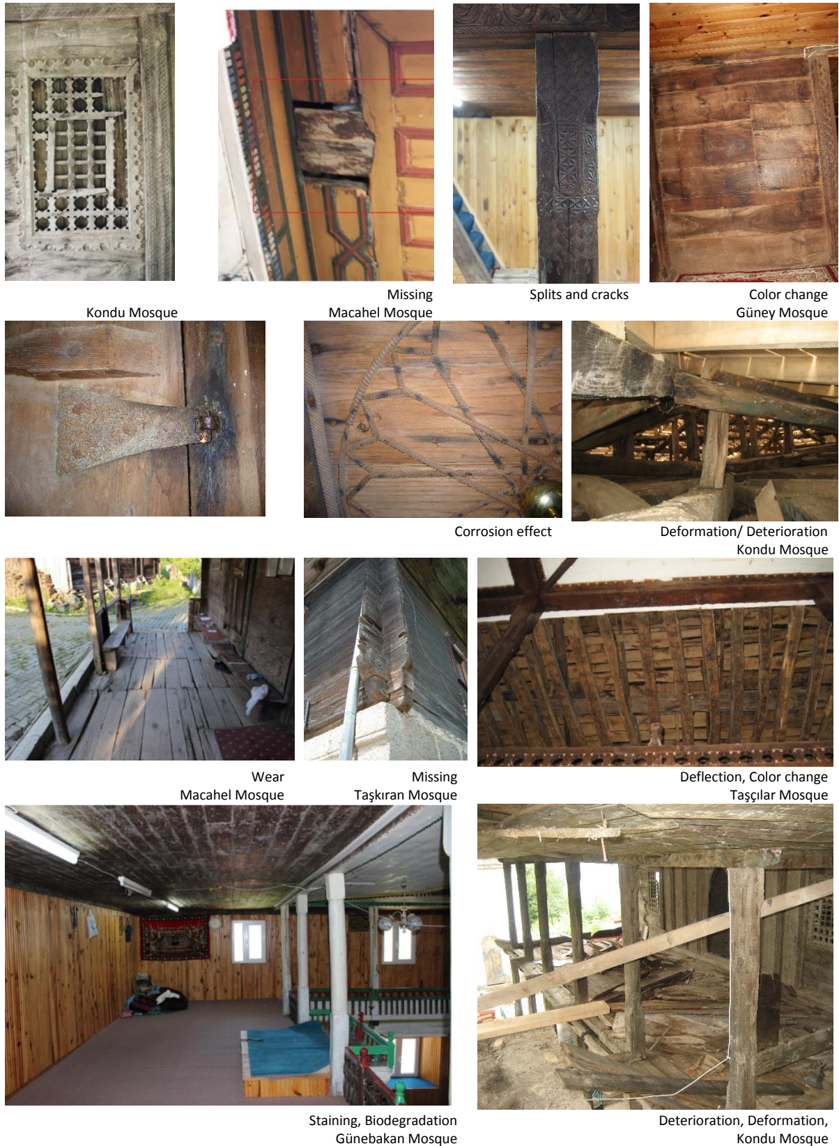
Figure 5. Examples of deformation in wood material originating from the environment in Wooden Mosques
